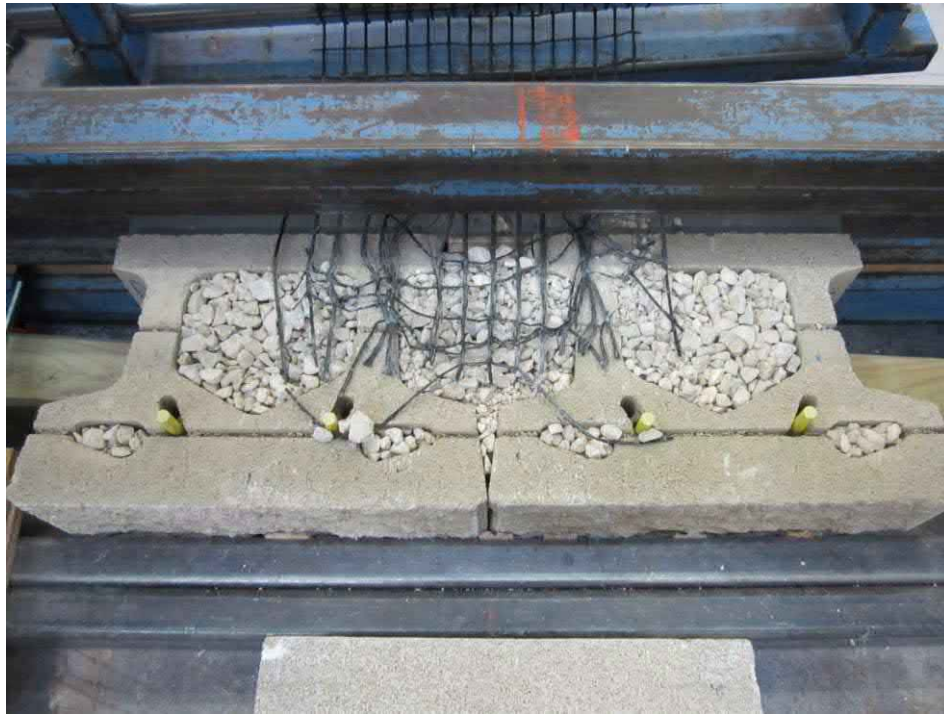
Figure 10: Photograph of exhumed grid specimen from Test 3 of index connection testing.
